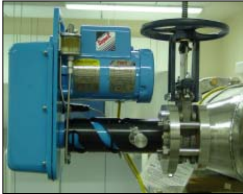
Figure 2. The rotating consistency transmitter installed through the gate valve.
